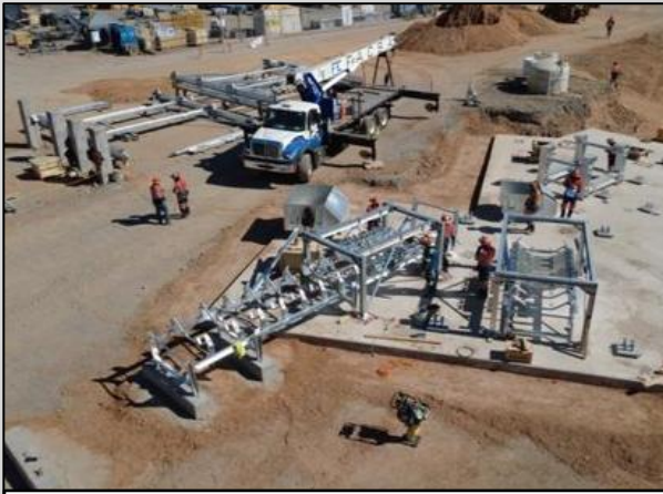
Assembly and installation of conveyor belt
