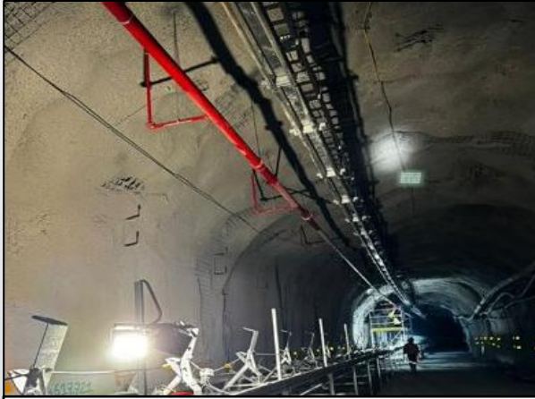
Installation of curved belt into Underground Ramp
