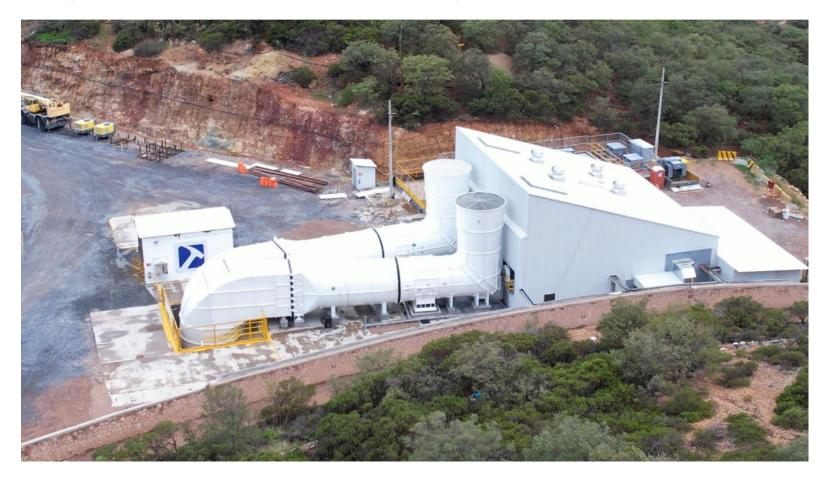
Two 2,000 horsepower ventilation fans installed at the surface of the Guadalupe shaft – a 5.5 metre by 580 metre deep, fully concrete-lined ventilation shaft
