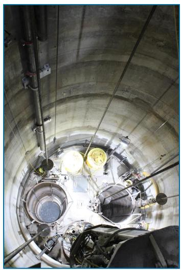
The fully concrete lined 5.5-metre diameter and 560-metre deep ventilation shaft is expected to be completed in 2023 at a cost of approximately \$47 million.
