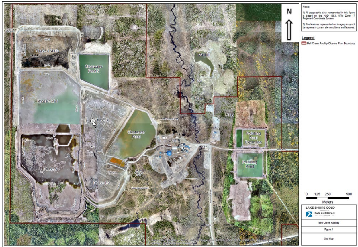
Figure 18.1: Bell Creek Surface Infrastructure
